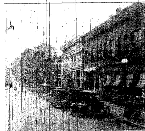
LOOKING WEST FROM MAIN
